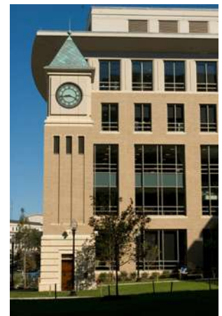
View of the Clock Tower and Wolff library
